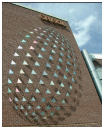
The front of the CREOL building that was completed early 1996.
